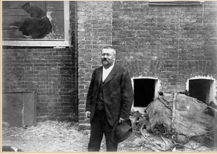
Savva Timofeevich Morozov at the construction site of the Moscow Art Theatre.
